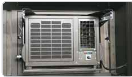
High performance air conditioning unit is used for heating and cooling of the living area. The air conditioner has a maximum cooling capacity of 4.9 kW which is performed as a combination of sensible and latent cooling. The air conditioner can adapt to ambient temperatures from -32° to +60°C.
