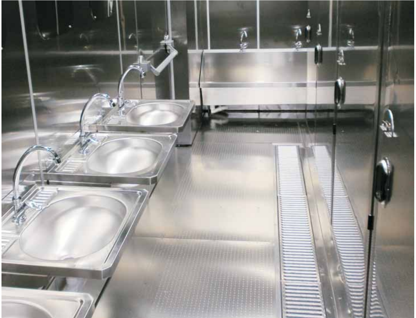
The configuration of 4 hole-in-the-floor toilets that has ability to become shower units by using the stainless steel shower trays , 4 sink units and 1 abluton unit fits in an insulated 20ft High Cube container which can cover all your sanitation needs.
